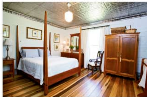
REFRESHER COURSE The poplar and heart pine floors were refinished throughout the house, including in the master bedroom (above), where Mark installed tin tiles on the ceiling. Top, in the eat-in kitchen, the brick chimney and plank walls keep the room rustic and true to its roots. A vintage-style stove complements the home's age.
